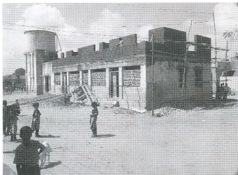
De schooluitbreiding in Pullicat is in volle gang.
